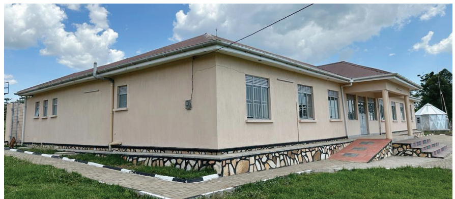
Namayingo Magistrate's Court was completed.
