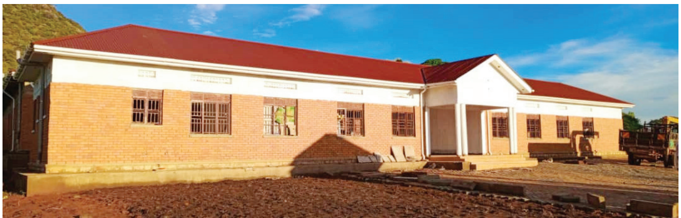
Karenga Magistrate's Court at the roofing stage.
