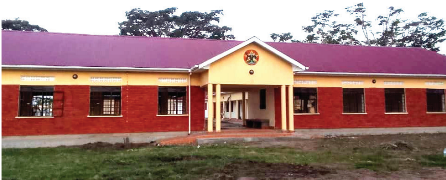
Patongo Magistrate's Court is at the finishing stage with painting and tiling works ongoing.
