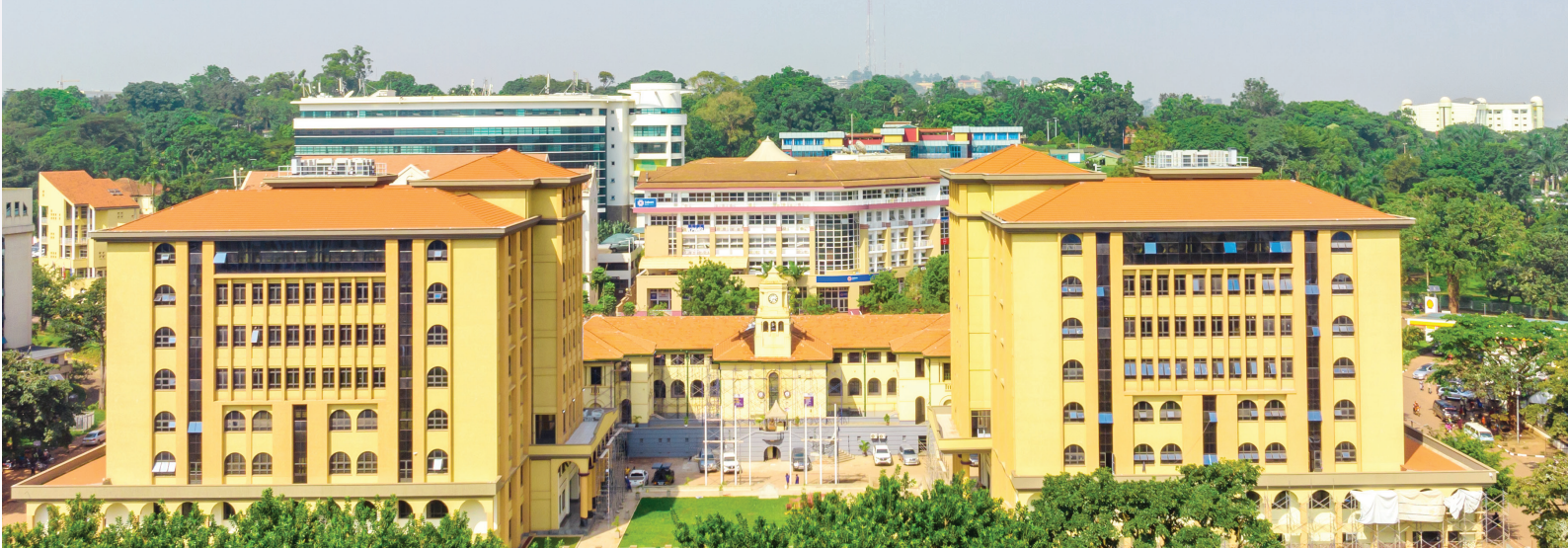
Above: The recently completed Supreme Court and Court of Appeal court buildings in Kampala.
